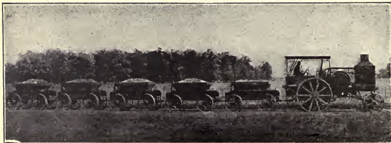
HAULING 22½ YARDS OF CRUSHED ROCK
